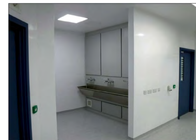
Scrub room with extract under trough
