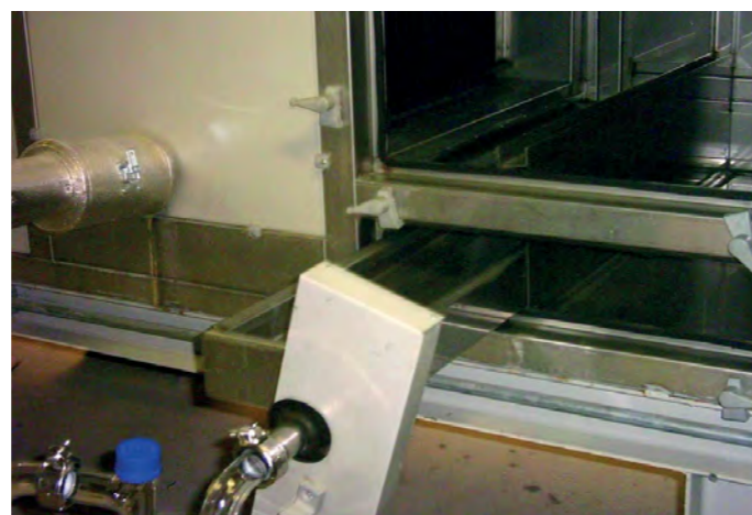
Removable AHU drainage tray
