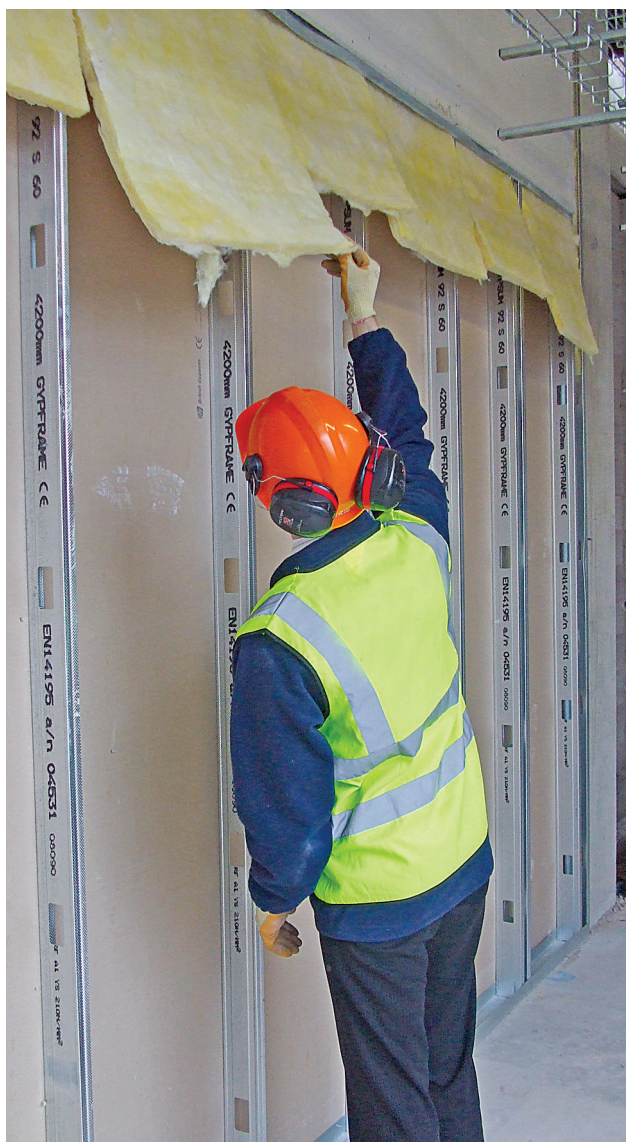
Site inspection (photograph courtesy of Sound Research Laboratories Ltd)
