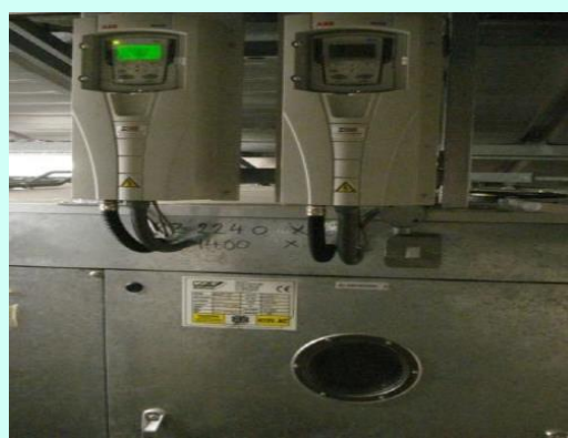
Figure 12 AC upgrades in the Barts Health NHS Trust included the installation of new energy filters (left) and VSD invertors on the AC plant (right). Courtesy of Barts Health NHS Trust
