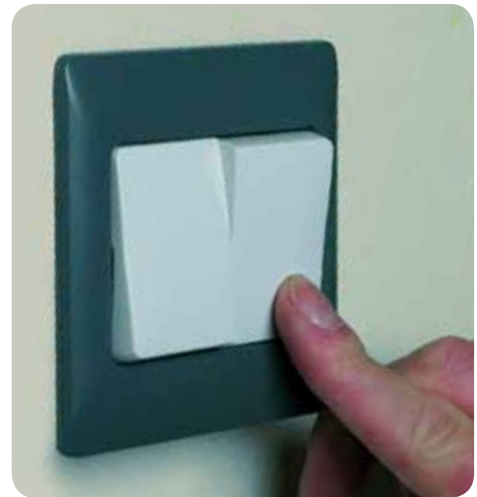
Photographs – Well contrasted rocker style light switches and sockets.
