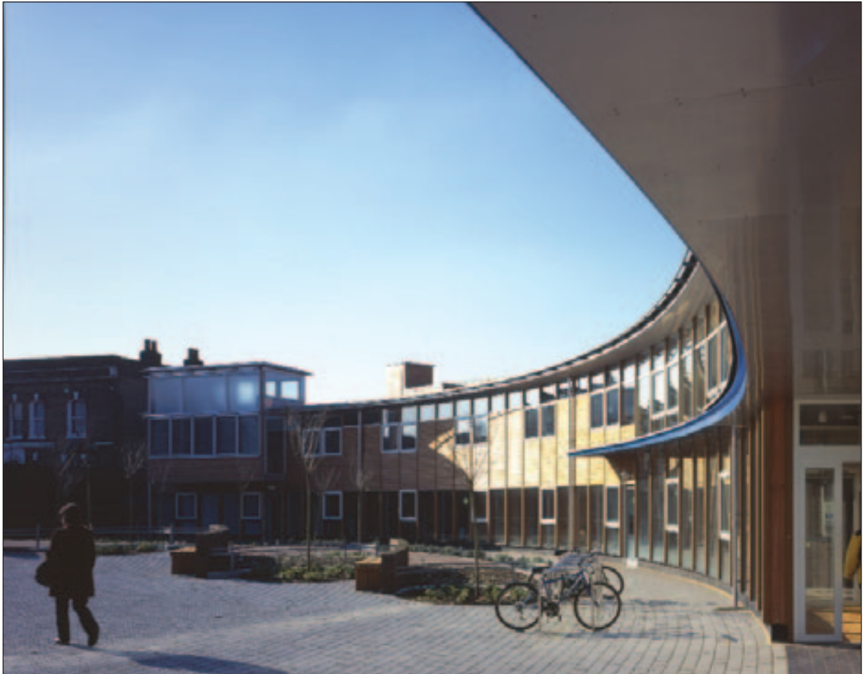
Front elevation, Pulross Intermediate Care Centre, London (Photo: copyright Marcus Peel)
