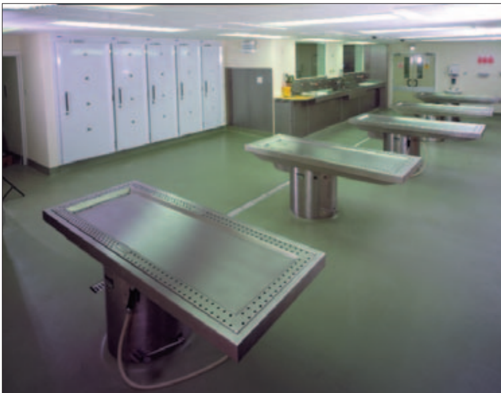
Post-mortem room showing down-draught ventilated post-mortem tables and pull-through fridges
