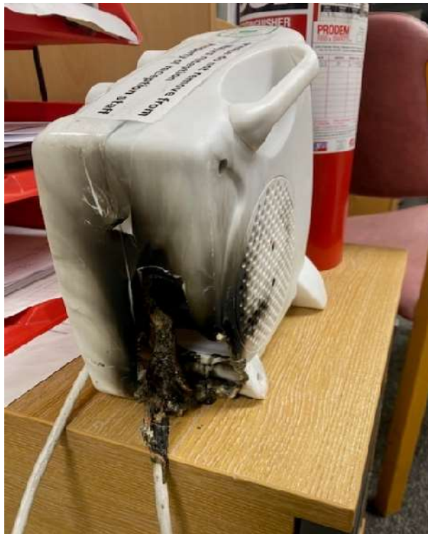
Figure 5 Example of an electrical-related fire involving a small portable heater, demonstrating the need to ensure equipment is appropriately tested, maintained, and used.
