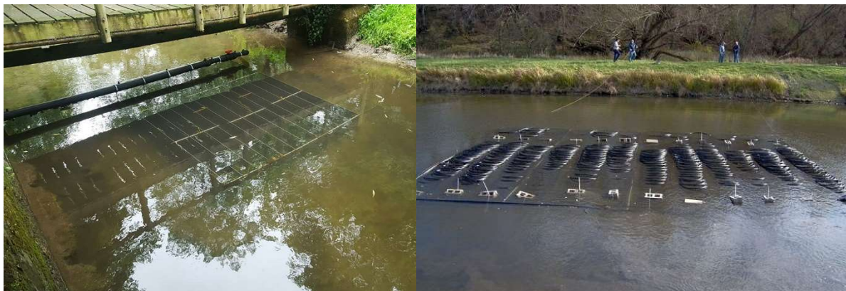
Figure 41. Outdoor heat exchanger coil installations for water source heat pumps 23
