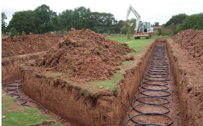
Figure 38. Installation of ground coils 21
