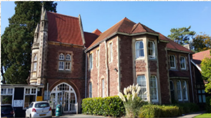
Rookwood Hospital, Llandaff, Cardiff
