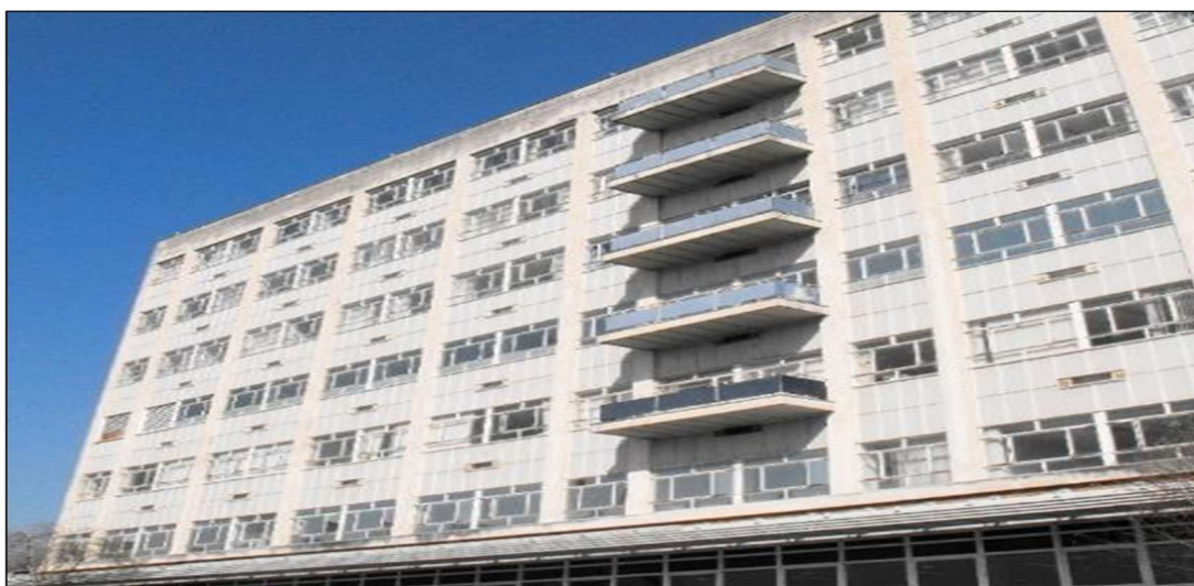
Original façade: Sash windows, crissal glazing and open balconies (source: SBUHB)
