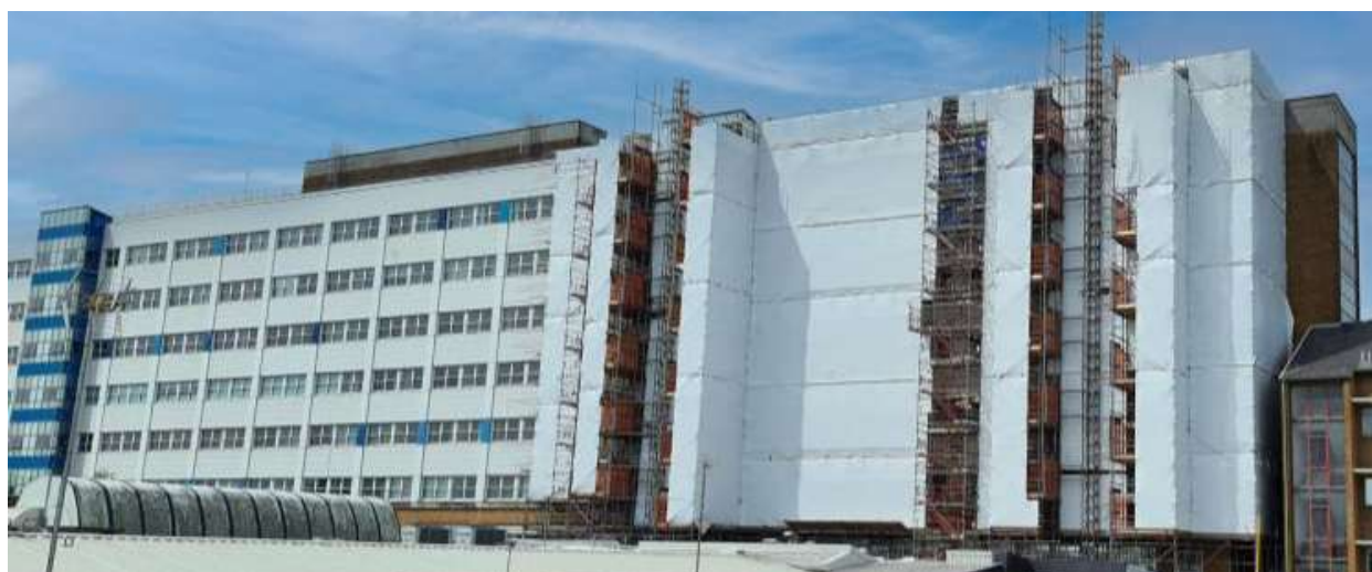
Main Elevation: Main contract: Works Phase 1 (source: SBUHB)
