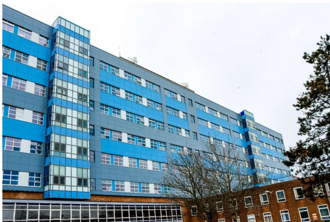
Main Elevation: New cladding installation with enclosed balconies (source: SBUHB)
