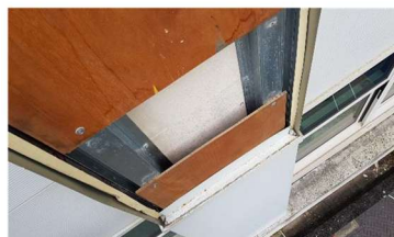
Plywood and foam insulation to column faces (main facade)
