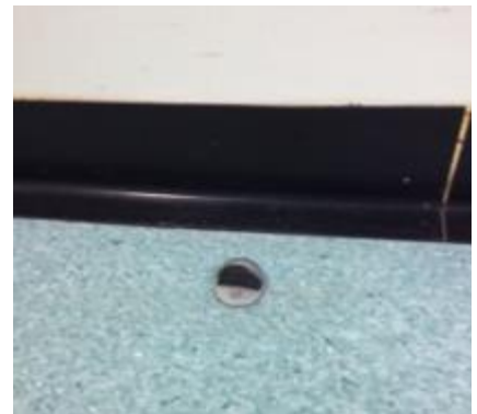
Figure 3: door buffer: ironmongery used to restrict door opening too far; fixed to either a door, floor or wall.
