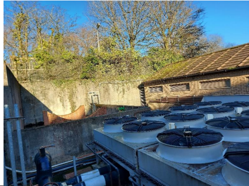
Photo 1 – Overview of the current land where the switch room is due to be constructed.
