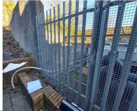
Photo 3 – Overview of the agreed placement of a secondary escape from the enclosed area.
