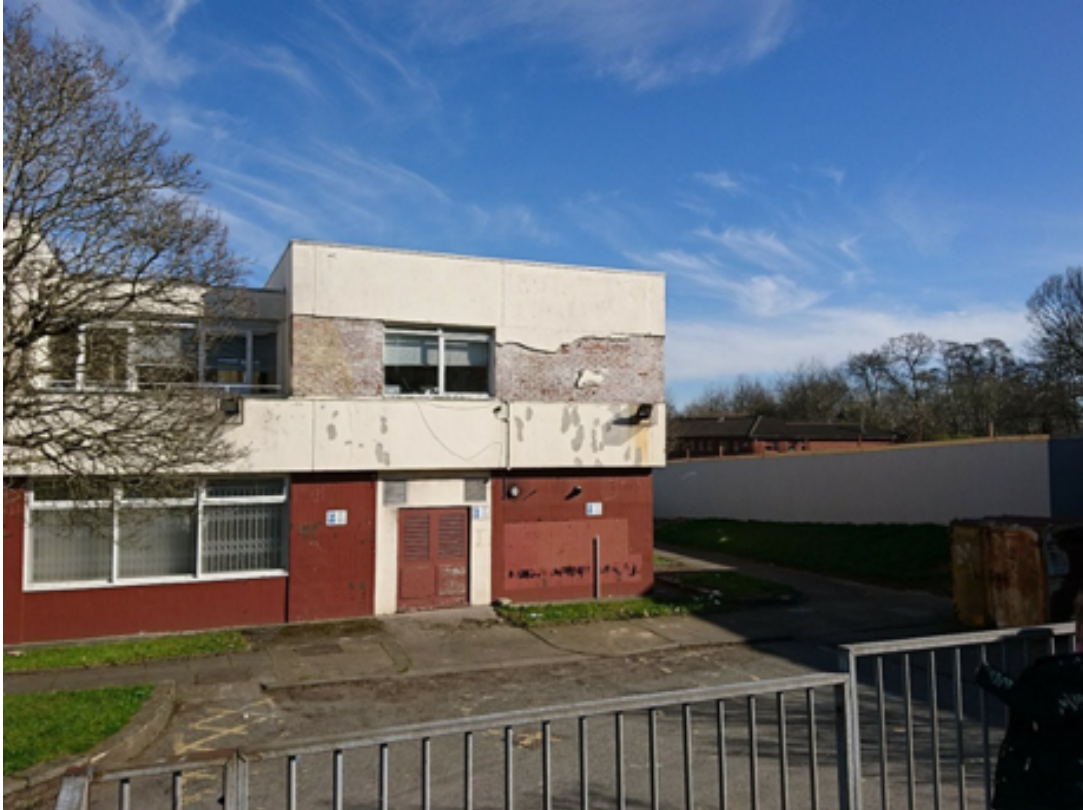
Figure 10: Existing external image of Llanedeyrn Health Centre
