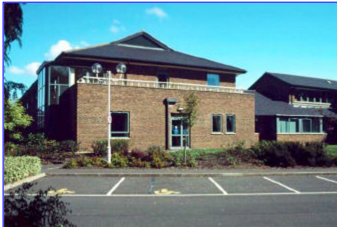
Figure 12 Chepstow Community Hospital
