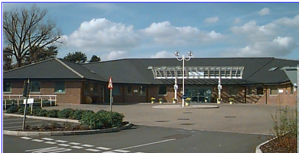
Figure 13 Chepstow Community Hospital
