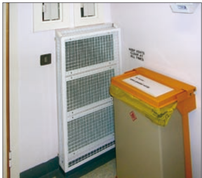
Pressure stabiliser with stand-off cage
