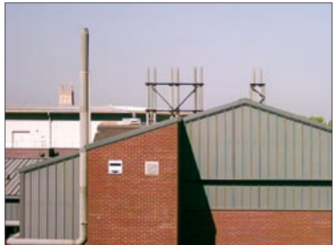
Typical LEV discharge stacks
