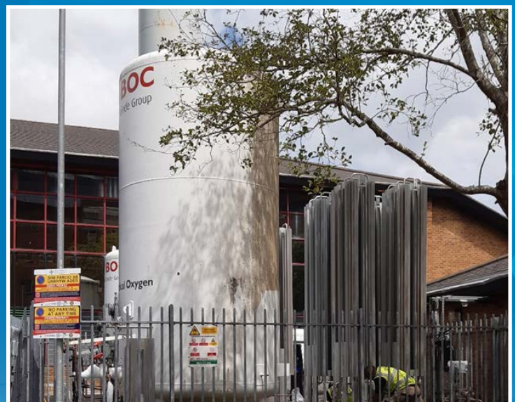
A Vacuum Insulated Evaporator (VIE) vaporiser upgrade in progress
