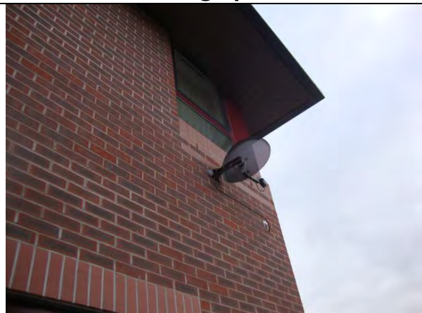
Dish in Place Photograph 60
