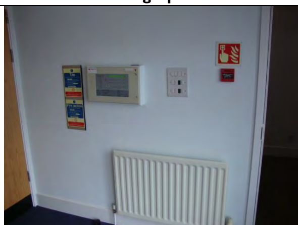
Ground Floor Lobby
