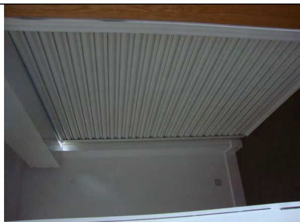
Ground Floor Shutter
